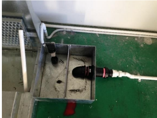
Gutter Box Plumbing and Float Placement
